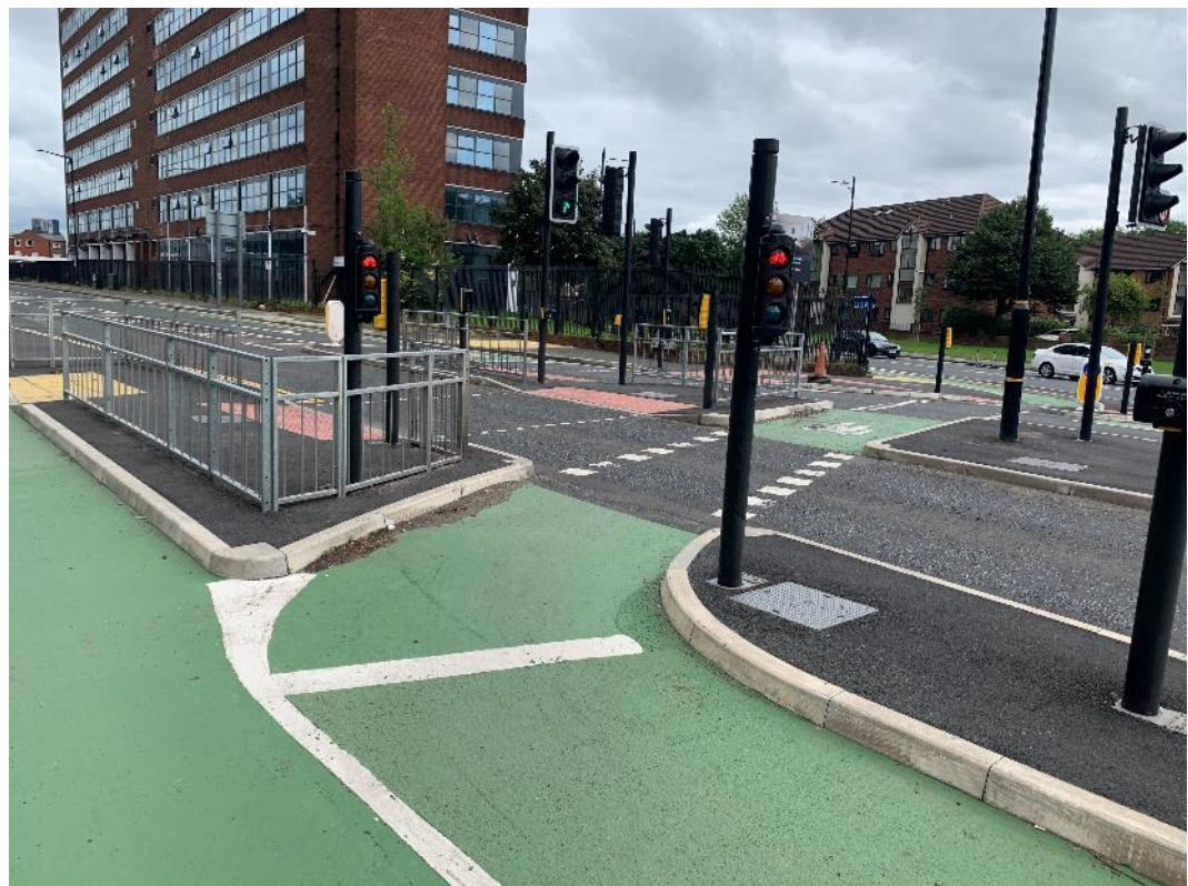
Figure 14: Protected right turn dedicated cycle phase, Trafford
