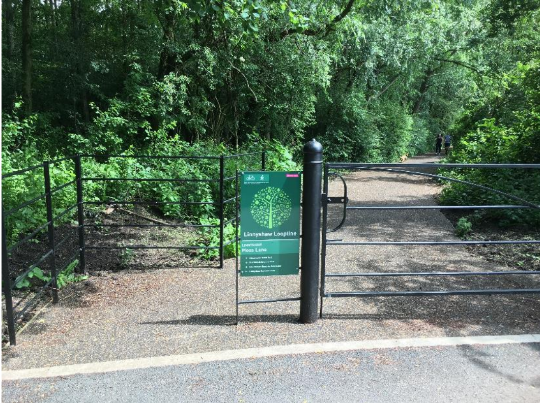
Figure 3: Accessible access control gate with lockable access for maintenance vehicles, Linnyslaw Loopline, Salford
