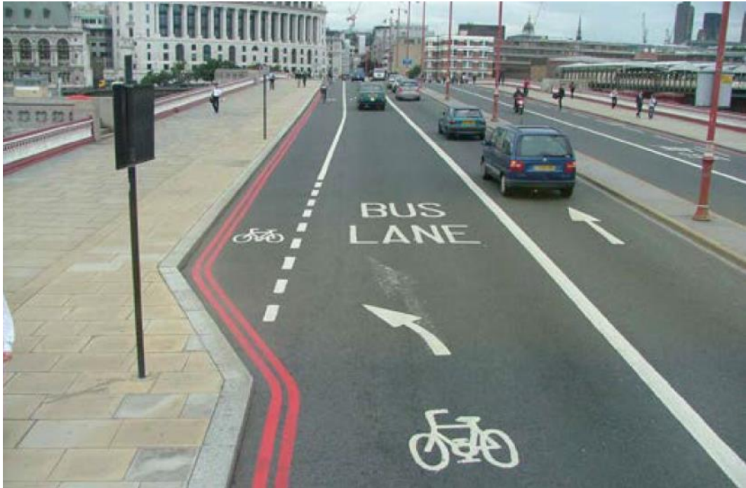
Figure 6: Cycle Lane within a bus lane (image reproduced from London Cycle Design Standards)
