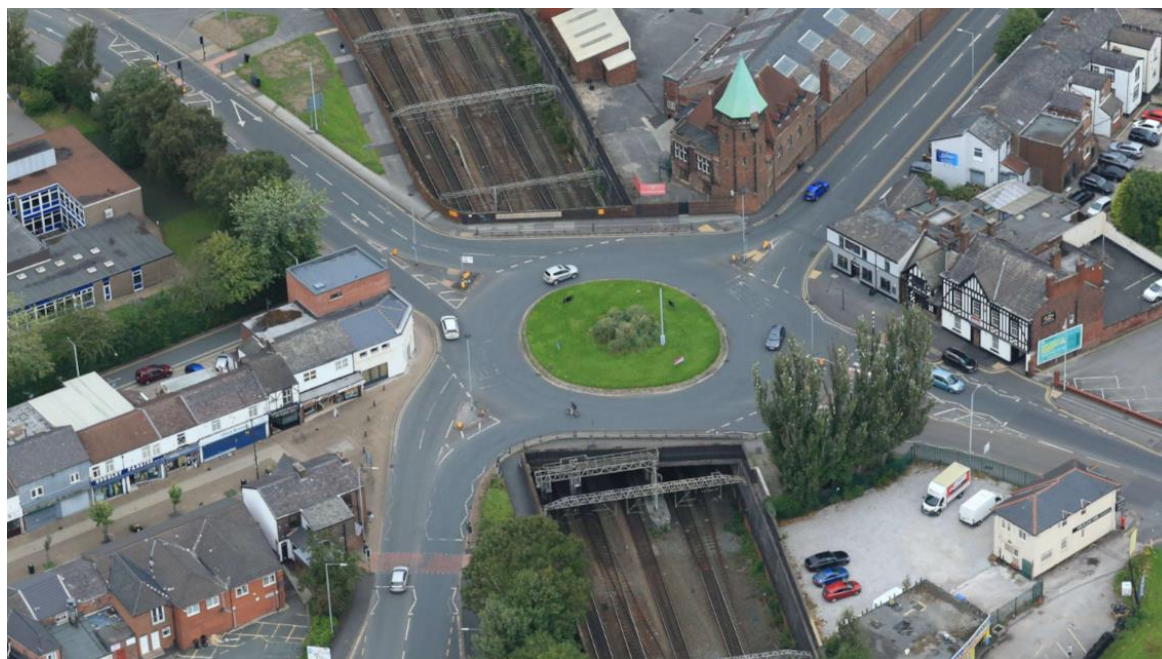
Aerial view of the existing Greek Street Bridge roundabout
