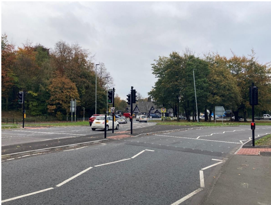
Salford, Worsley Brow: Puffin crossing and permanent traffic signals installation
